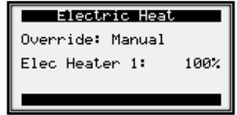
Figure 5 - Electric Heat Override Page. Set override to manual and set to 100% to complete startup.
